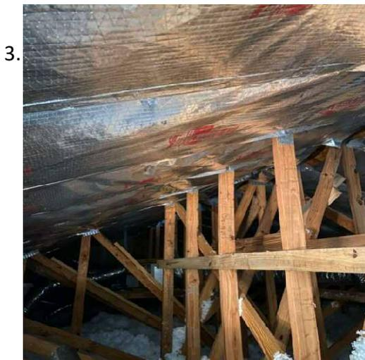
3. Leak sourcing. Since the existing roof runs seamlessly over all of the Villas in each building, it may be possible for an owner to replace his/her roof, only to find the source of the leak to be from a neighboring roof. Those Villas with “radiant barriers” (see photo to left) installed under their roofs, in their attics, also exacerbate leak sourcing. Replacing the entire building roof at one time should eliminate this potential problem.
